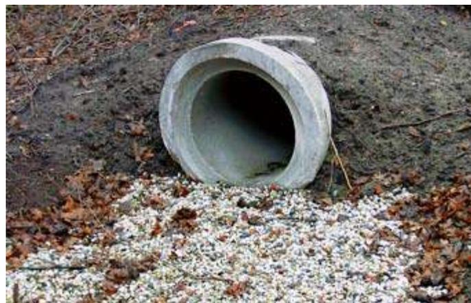
**Figure 33 Gravel pit removes water well** (den Ouden & Piepers, 2008)
