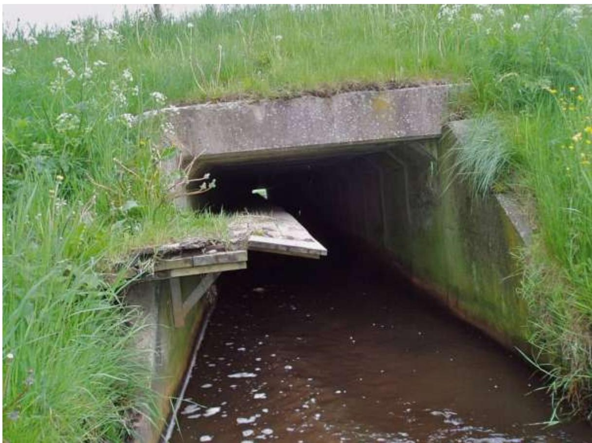
Figure 26 Poorly maintained mammal ledge in a culvert (Photograph: H. Bekker)
