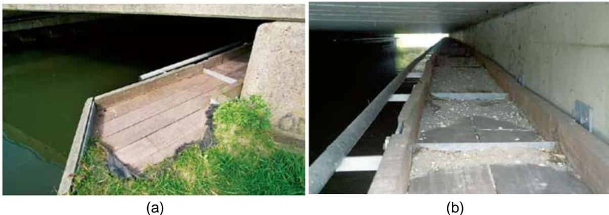
Figure 27 (a) Good connection to the shore (b) Missing sand layer (den Ouden & Piepers, 2008)
