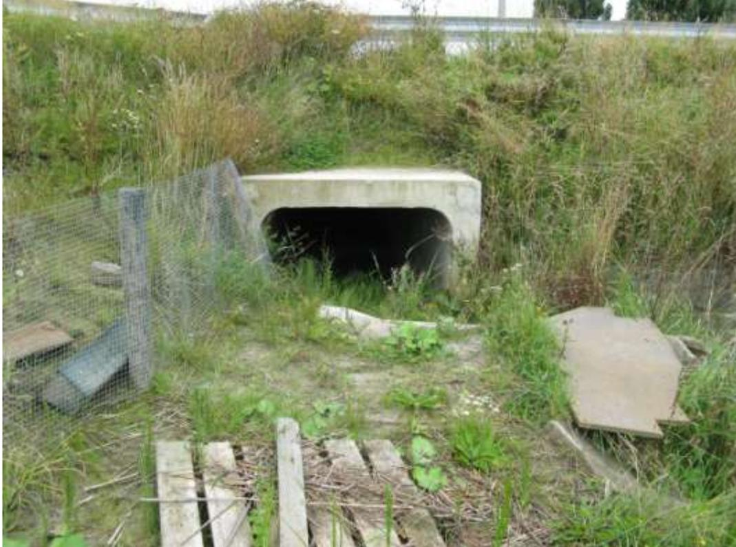
**Figure 31 Culvert with rubbish and construction materials strewn around the entrance (Wansink 2013)**
