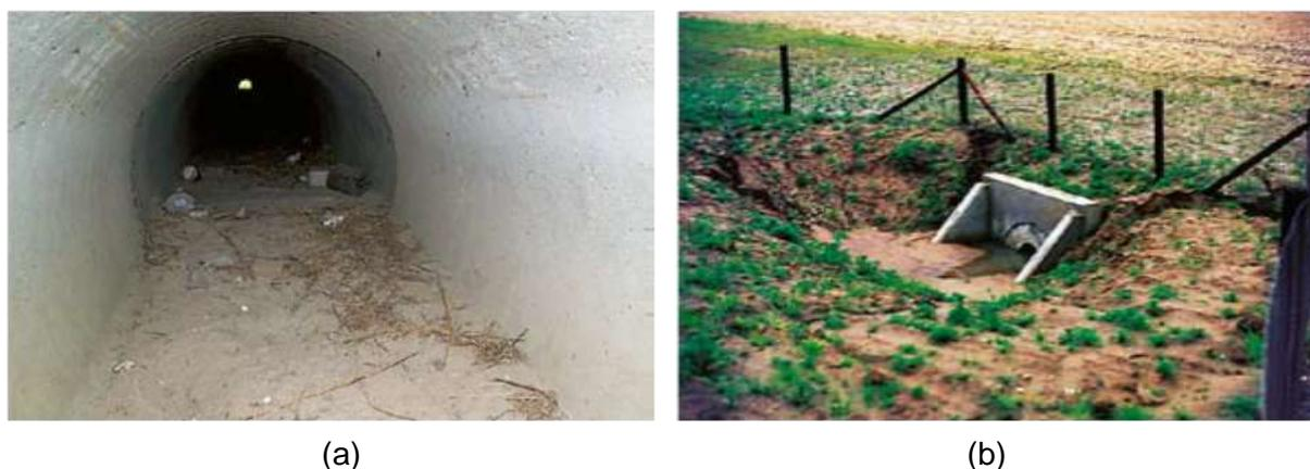
Figure 30 (a) Tunnel easily accessible, free of obstacles (b) Tunnel full of water (den Ouden & Piepers, 2008)
