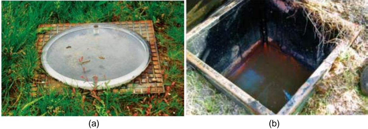
**Figure 32 (a) Accessible and well sealed (b) Inspection vent full of water** (den Ouden & Piepers, 2008)
