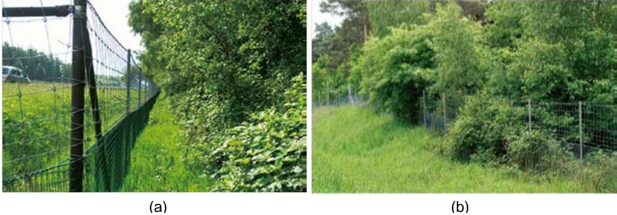
**Figure 14 (a) Easily accessible for inspection (b) Vegetation overgrown through fence** (den Ouden & Piepers, 2008)
