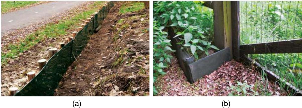
**Figure 5 (a) walkway is easily accessible (b) walkway (right of screen) is overgrown, escape is possible.** (den Ouden & Piepers, 2008)
